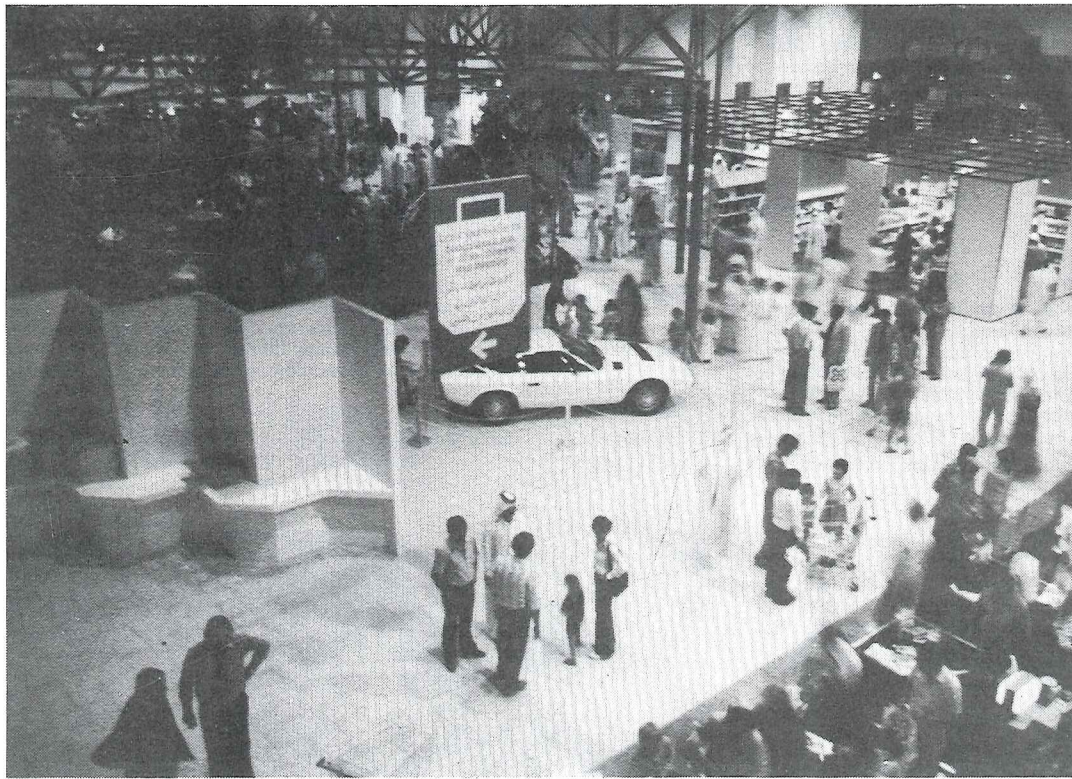
Doha Centre which was completed in thirteen months.
